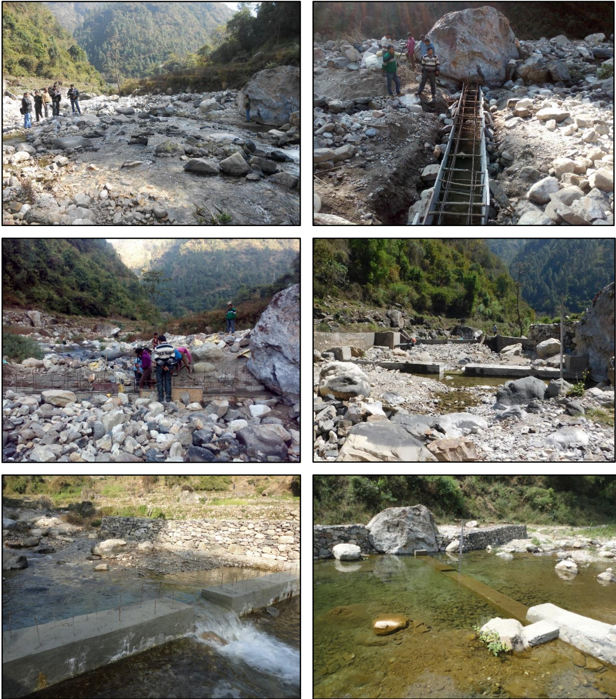
Fig. 3. 2 Various phases of construction of Weir at Jijali
