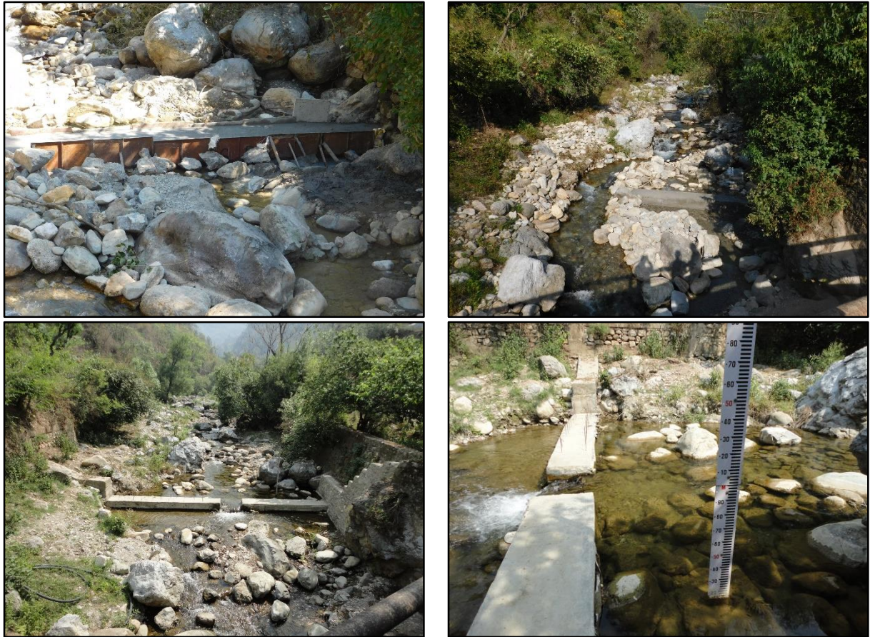
Fig. 3. 1 Various phases of construction of Weir at Herval
